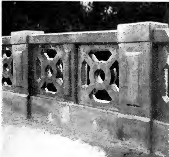
Fence comprises pre-cast newels, panels and coping.
